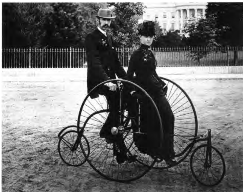
A cycling couple posing in front of the White House, about 1885. Tandem three- and four-wheelers were then popular with affluent couples who were determined to cycle together. This one could be converted into a single tricycle by loosening bolts in the center and detaching either the front or the rear portion.
