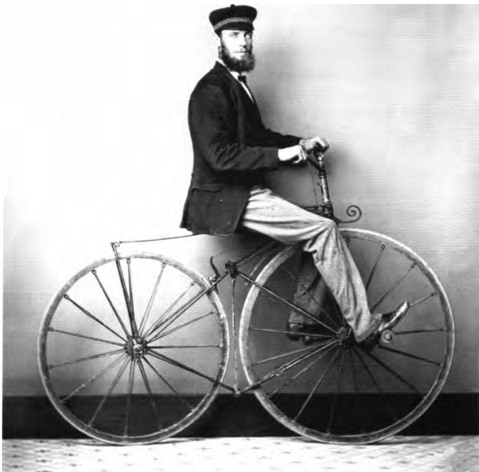
An unidentified New Zealander proudly poses with his Phantom bicycle, about 1871. The Phantom Wheel Company of London exported its distinctive bicycle with the unique pivoting frame around the world and won a small but devoted following. Nevertheless, the high wheel continued to gain favor and the company folded in the fall of 1872.
